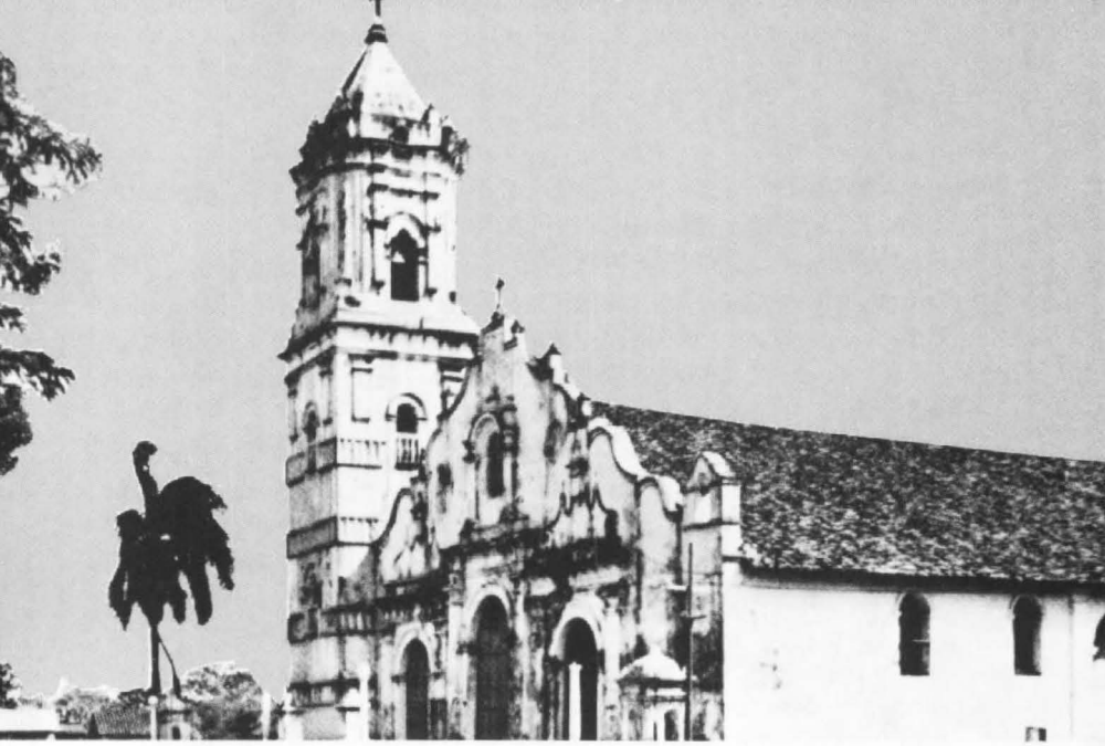
Church of Natá, built in 1522; believed to be the oldest church still in use on the mainland of the Americas
